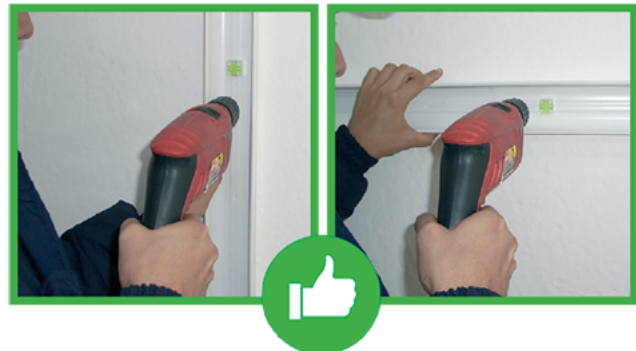
Duct installation with built-in level
