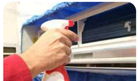
Battery cleaning without protective cover
