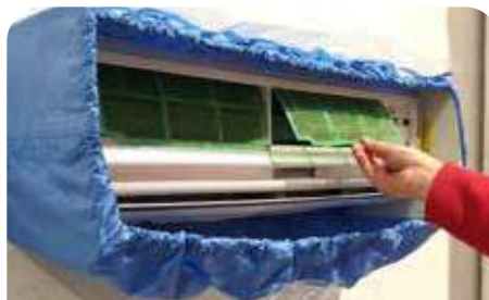
Removing the filters
