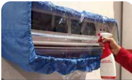
Battery cleaning with protective cover
