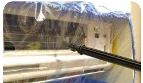
Battery cleaning through cleaning machine hole
