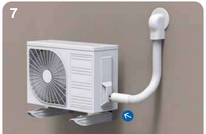
Flare the refrigerant pipes and fix them to the taps of the outdoor unit, connect the power supply. Approach and position the rubber sleeve near the taps
