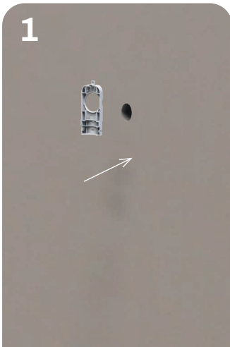
1 Fix the rear part of the aesthetic flange in correspondence with the wall hole
