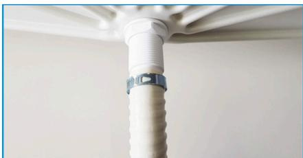
INSERIRE IL TUBO SCARICO CONDENSA COIBENTATO E FISSARE IL TUTTO CON LA FASCETTA STRINGITUBO. / INSERT THE CONDENSATE DRAIN PIPE AND FASTEN EVERYTHING WITH THE HOSE CLIP.
