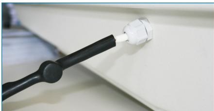
FAR SCORRERE IL CAVO SCALDANTE NEL PASSACAVO FINO ALLA BATTUTA DELLA GUAINA DEL TERMOSTATO E BLOCCARLO. / INSERT THE HEATING CABLE THROUGH THE GLAND-NUT TILL THE THERMOSTAT AND FASTEN IT.
